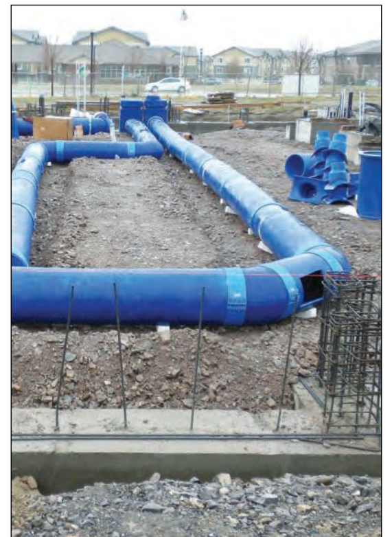
PLASTIC DUCT READY TO BE INSTALLED AT A PROJECT SITE – PHOTO COURTESY OF AQC INDUSTRIES.
