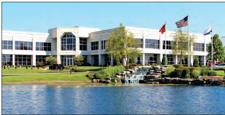
A.O. SMITH'S LEBANON, TENNESSEE MANUFACTURING FACILITY.
