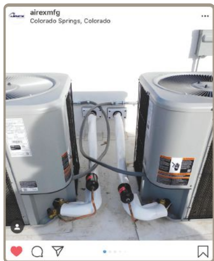
Commercial - RoofTop Install
