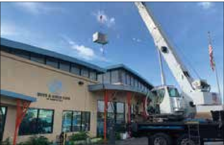
Quality Refrigeration prepares to install a package heat pump at The Boys & Girls Clubs of the Los Angeles Harbor facility.
